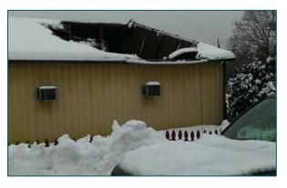
The most hazardous conditions are likely to arise when repeated snow falls, that can take place over several days, do not have sufficient time to melt from roofs that can consequently accumulate and exceed the design capability of the roof. Furthermore, conditions can be exacerbated when rain follows heavy snow falls as rainwater will initially be absorbed by the snow layers which will further increase the weight of the snow layer.
