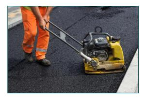
Hand-arm vibration is vibration transmitted into workers' hands and arms. This can come from use of hand-held power tools (such as grinders or road breakers), hand guided equipment (such as powered lawnmowers or pedestrian controlled floor saws) or by holding materials being worked by hand-fed machines (such as pedestal grinders or forge hammers).
