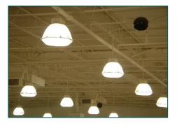
plasma greatly increases the intensity of visible light produced by the arc for a given power input, as the metals have many emission spectral lines in the visible part of the spectrum. HID lamps are a type of arc lamp.
