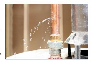
**Heating and Cooling systems.** Boiler equipment, filtration plant, water tanks, air conditioning systems etc., can all cause water damage if not properly maintained or as a result of faults.
