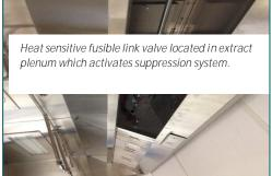
The fire suppression system should be designed and installed by an engineer with third party certification, such as the <u>BAFE Kitchen Fire Suppression Systems Scheme SP206</u> covering the design, installation, commissioning, recharge and maintenance of kitchen fire suppression systems from an independent UKAS accredited third party certification body.
