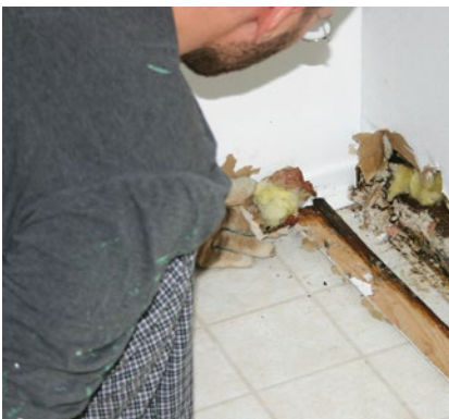
Step 4 Reinstall all damaged areas
