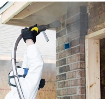
Step 4 External restoration works
