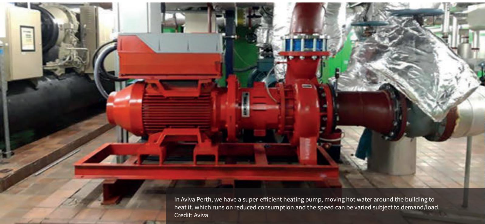
In Aviva Perth, we have a super-efficient heating pump, moving hot water around the building to heat it, which runs on reduced consumption and the speed can be varied subject to demand/load. Credit: Aviva
